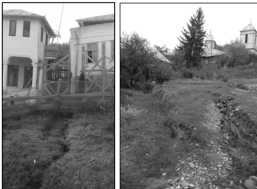
Fig. 6. Landslide in Rătești – October 2014.
